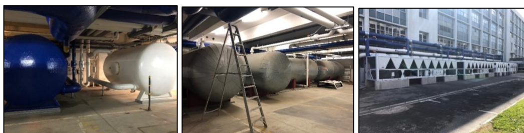
Phase II installation of Tygerberg campus's central HVAC system (from left): the central chiller plant, buffer tanks and water storage tanks.
